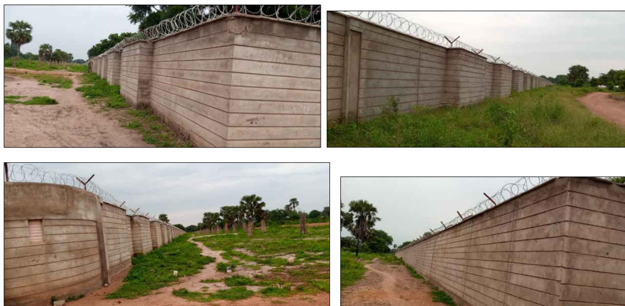
Photos: Different Sections of the complete Plastered, coped Loreto Security Wall with Razor Wire.
