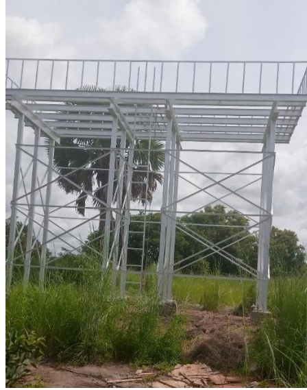
Above: Left Water tank installed at the school farm (Green house at the background), Right, water tower construction in progress awaiting installation of tank.
