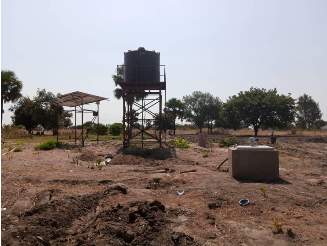
Photo: The school farm water tower system showing the solar powered water pump
